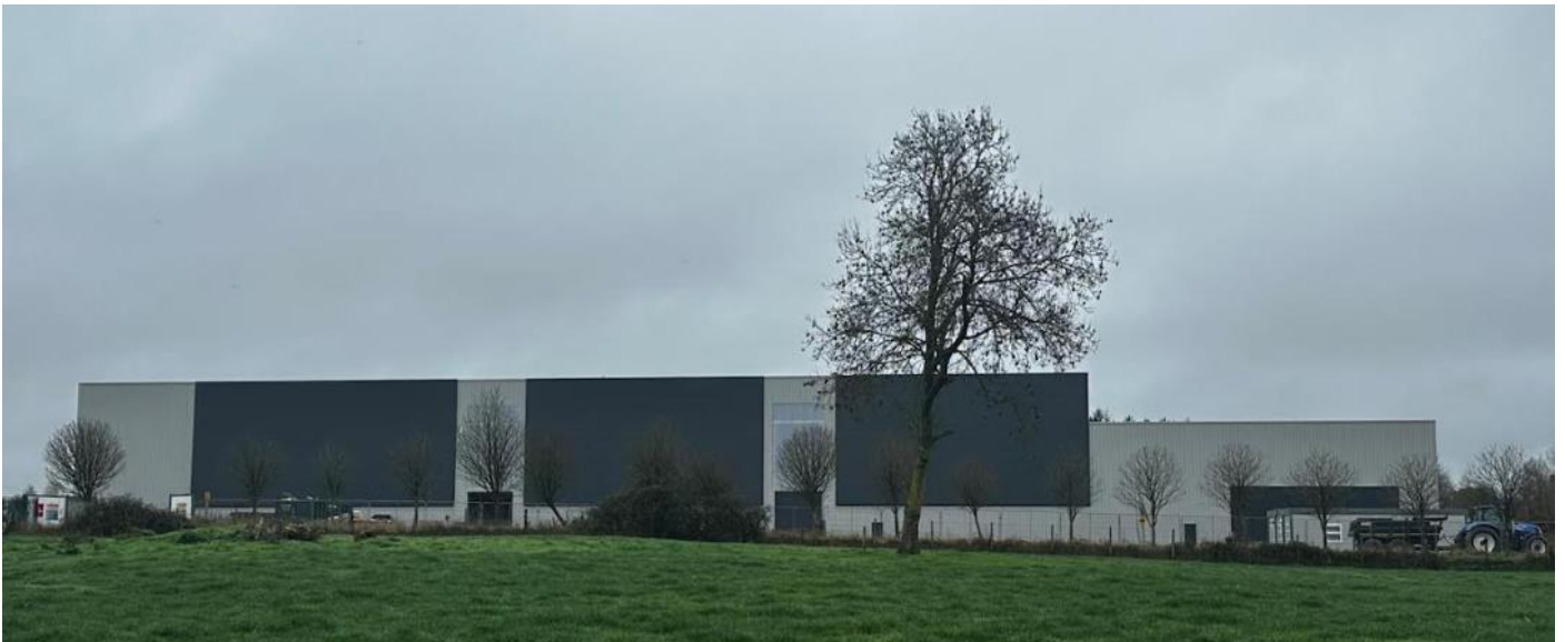
Figure 1- Photo of front facade as completed
